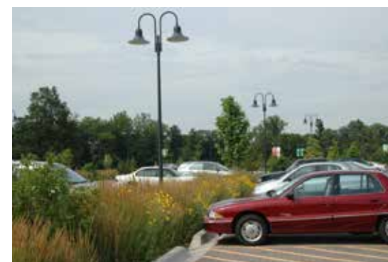
Bioretention areas integrated into parking lots can help slow and treat stormwater
