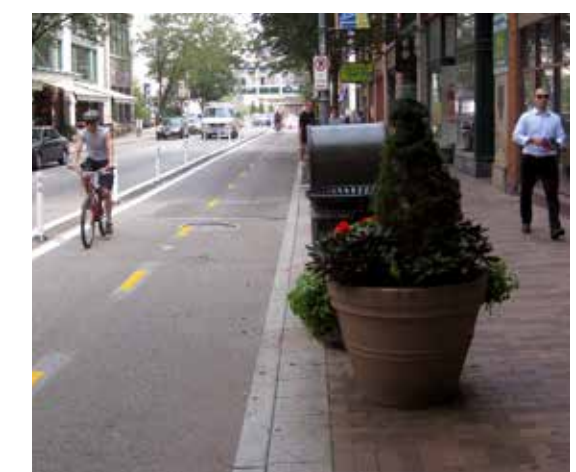
Two-way bicycle path created from a single vehicle travel lane
